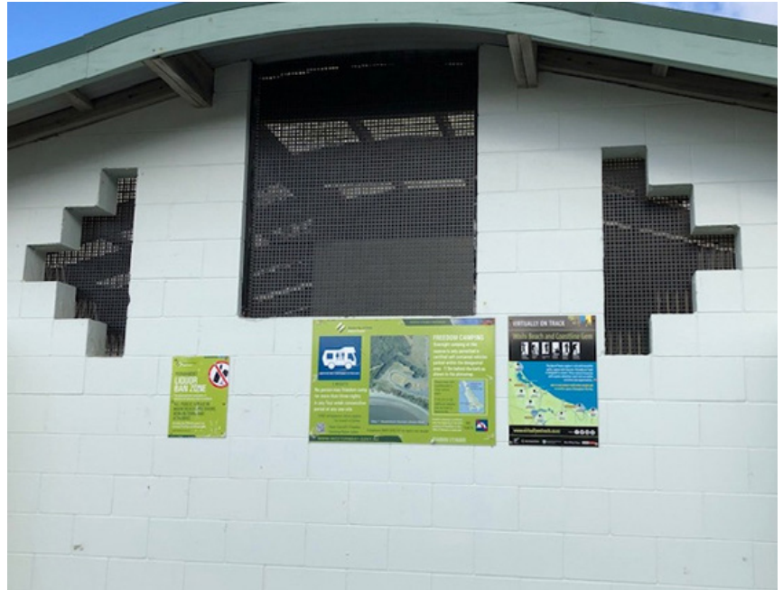
Discreet grating finish allows light and airflow while blocking bird entry.
