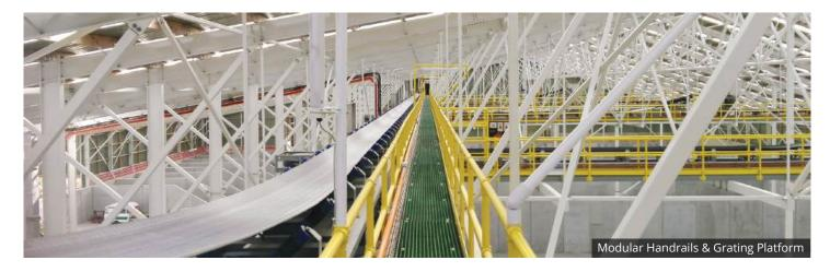
Our FRP grating, anti-slip products, and modular handrail and guarding systems are ideal for many industrial applications, including hazardous environments. They are durable, easy to install, low maintenance, and highly resistant to slips, fire, and corrosion. Without the lead times typical with steel fabrication, our handrails and guarding eliminate the need for on-site formalities like hot work permits.
